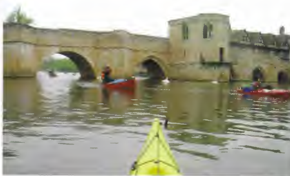
Above: The 14th Century bridge with chapel in St Ives.
