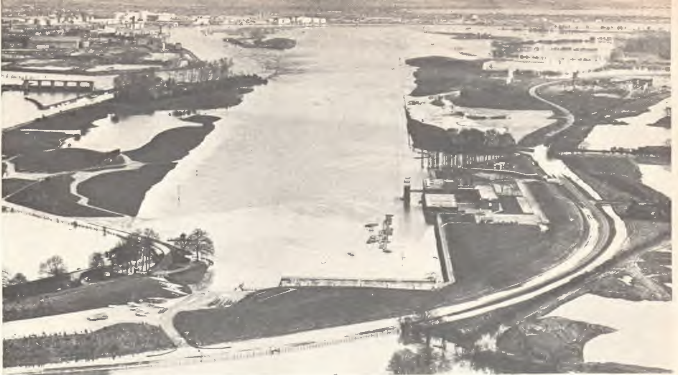
The National Watersports Centre, Holme Pierrepont, at the height of the floods and as you've seen it all before! Note water streaming over on to the course at the lower lefthand and top lefthand. The fine line running up the course on the right and just in front of finish tower is the lamp standards protruding from the water!
