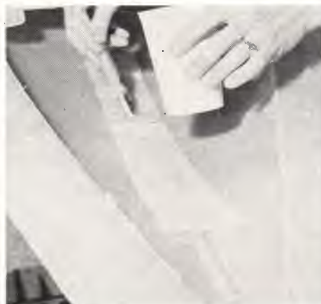
Glassing keel dowel in position
