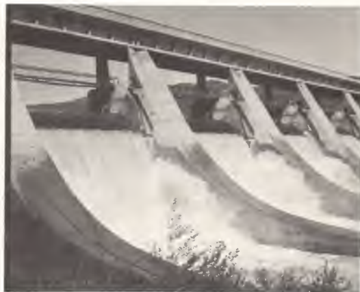
Dam at Chateaux Arnoux
