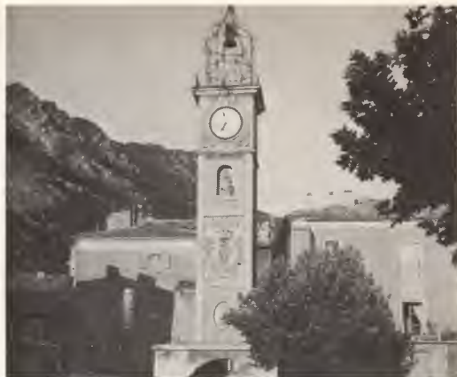
Old Tower in Sisteron .
