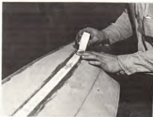
18. Outside joints being taped.
