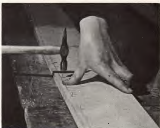
6. Fixing the inwales in place.
