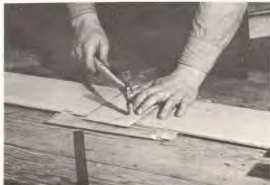
2. Making the butt joints on bottom panels.
