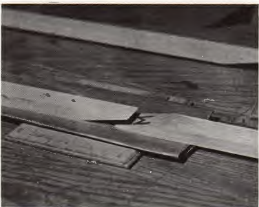
5. Making scarf joints on the inwales.
