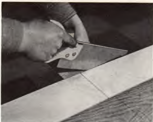
3. Trimming butt joints.
