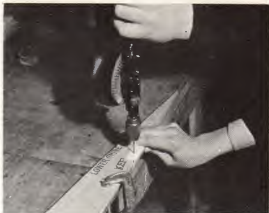
4. Drilling holes for lacing.
