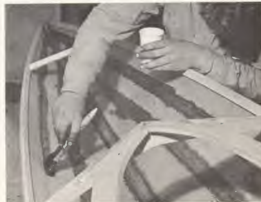
16. Inside joints being taped
