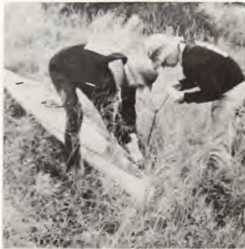
Repairs at Campbells Farm.
