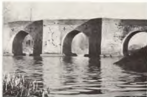
Yalding Road Bridge.
