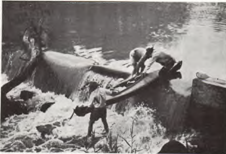
Typical obstacle—one of the many weirs on the upper reaches
