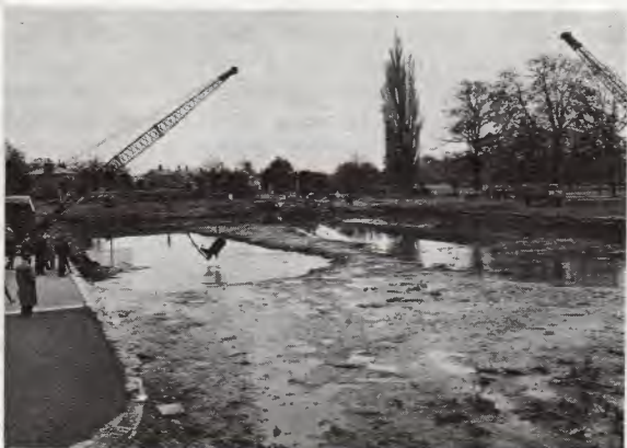
19 RB's of Western Command Plant Troop dredging from sides of canal basin.
