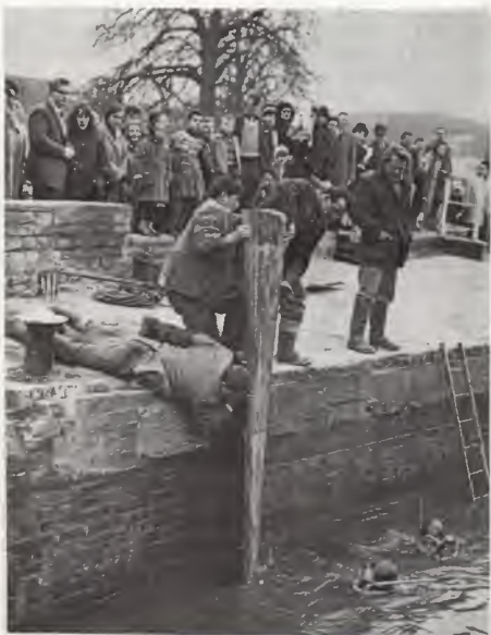
Frogmen clearing away lost obstacles in lock 56
