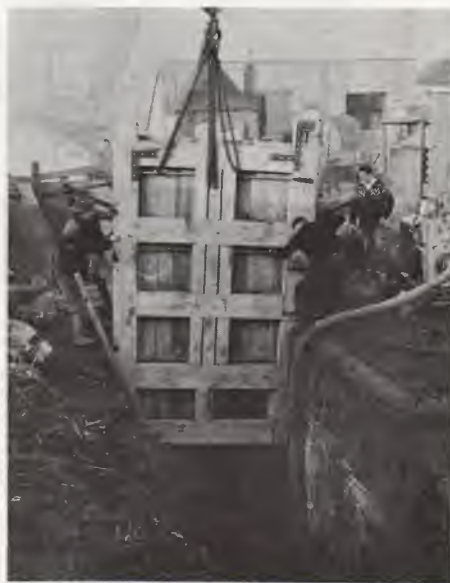
First lockgate being installed by Army Crane
