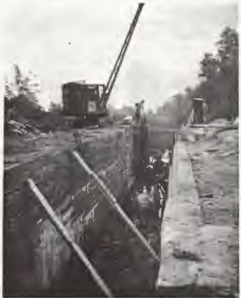
Removing demolished wall and mud from lock 43. Wilmcote flight. Summer 1963.
