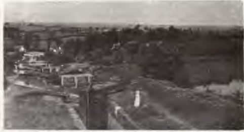
Foxton Locks. The old incline lift was on the right.
