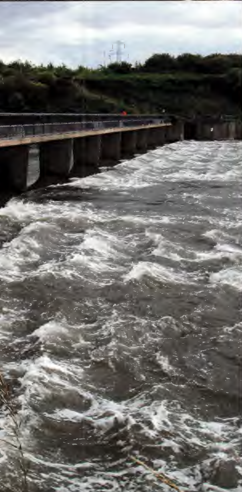
The Teesside International White Water Centre has some great features
