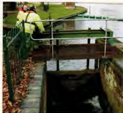
Above: Environment Agency Operatives get ready to "Pull" the Duck Mill Sluice.
