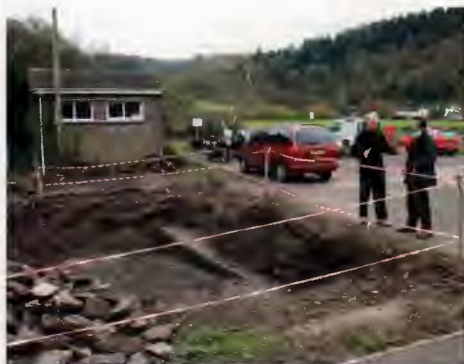
Above: The partially uncovered Roman slipway at Fryer's Wharf Tintern, the River Wye is behind the pumping station.
