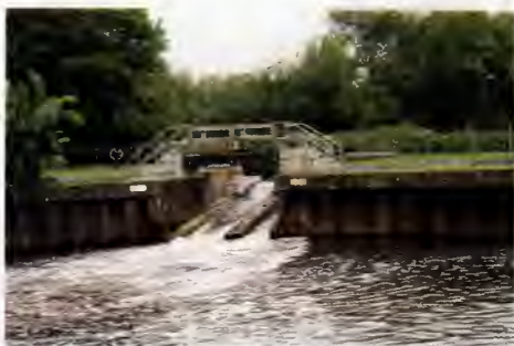
Above: East Lock Canoe and Fish pass looking up stream.
