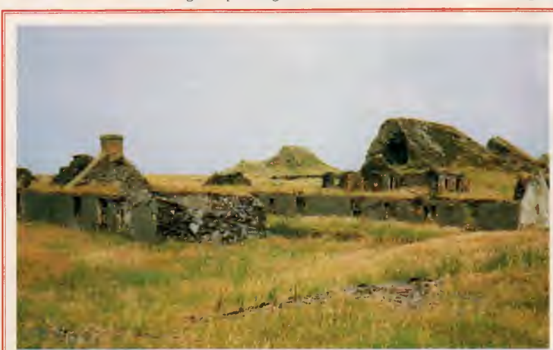
Above: Former mining settlement in Belnahua. Below: Mike Hart off Jura.
