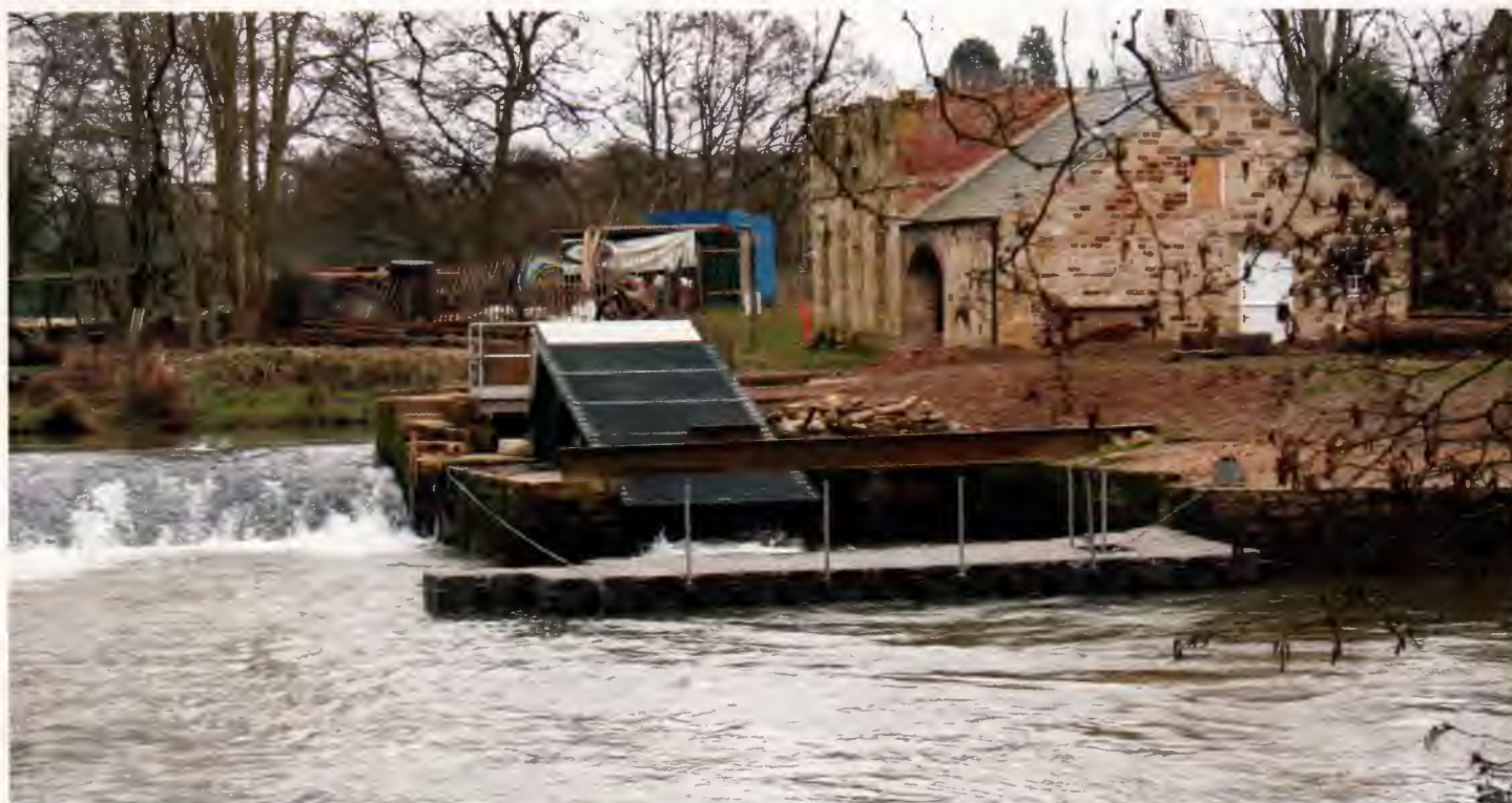
Above: Howsham Weir on the Yorkshire Derwent near York in medium water conditions. Though difficult to see the turbine below the mesh, it is taking more than 50% of the river flow.
