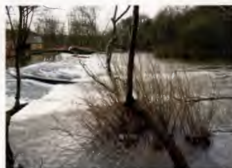
Above: Howsham Weir showing the canoe slot installed in the late 1980s with Sport England money to facilitate slalom. The hydro screw in the distance at the opposite end of the weir. The flow through either affects the other and the weir is a shadow of its former self.
