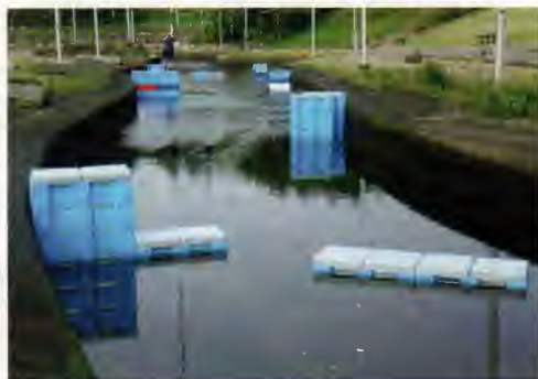
Above: Rapid blocks in place at Teesside.
