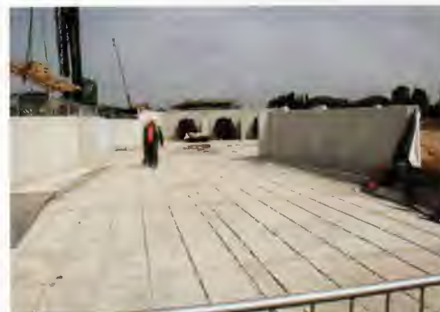
Above: Broxbourne under construction.
