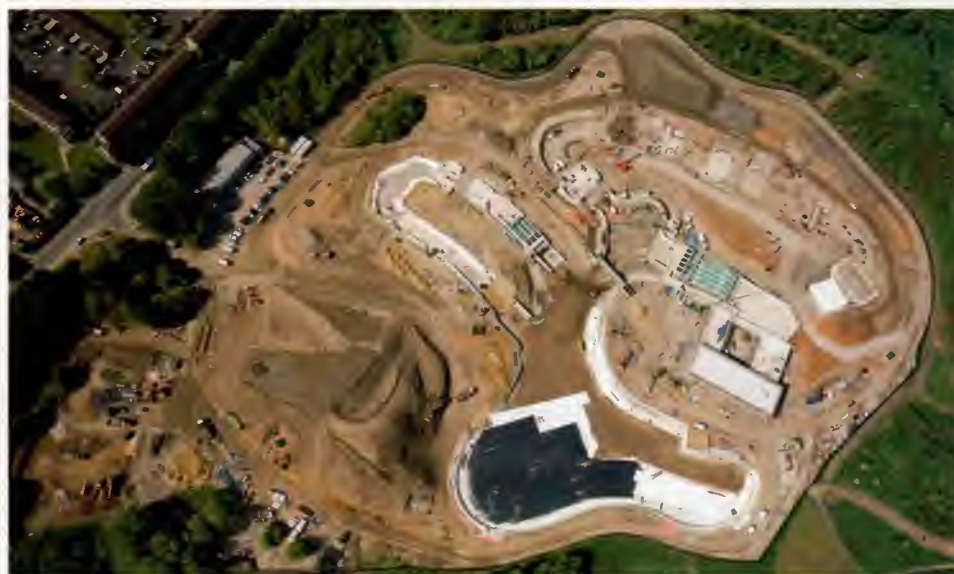
Above: Top aerial view of the site showing the progress.
