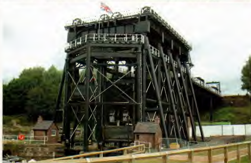
Above: The refurbished Anderton Boat Lift.
