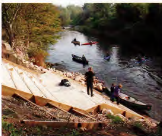
Above: Heaton Mersey ingress. Photo: Chris Hawkesworth.
