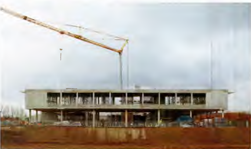
Above: The facilities building.
