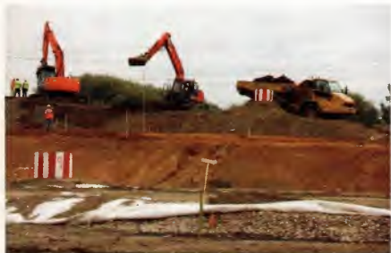
Above: Construction at Broxbourne.
