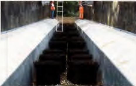
Above: View of the fish brushes and after completion at Allington Lock.
