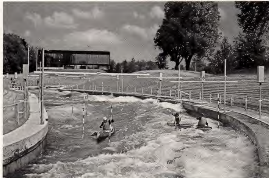
Augsburg, West Germany, The first artificial Olympic Slalom Course — built in 1972
