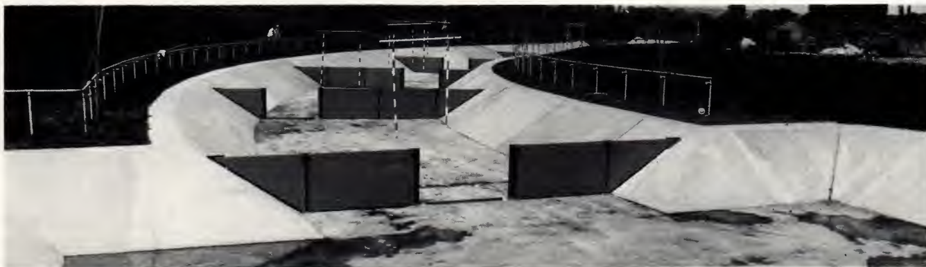
The course with barriers in position prior to opening the sluice gates
