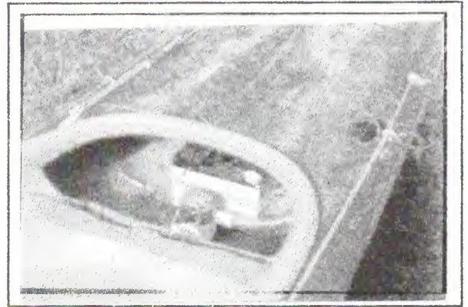
This shows the battery and pump, and the outlet (a 900 polypipe fitting)
